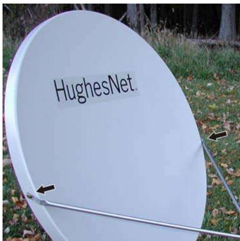
Figure 16: Attaching support rods to the reflector
