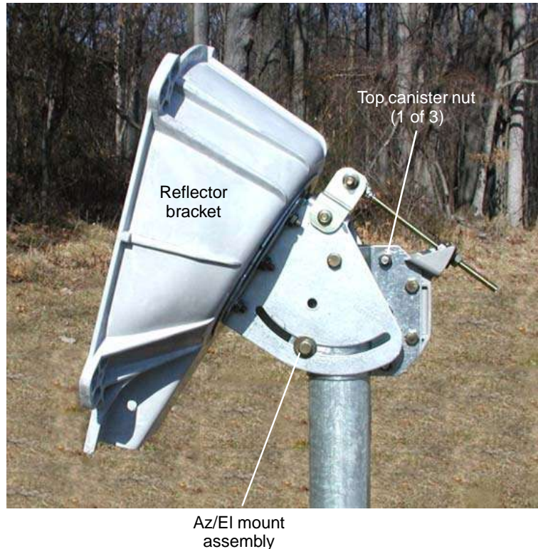
Figure 22: Az/EI and reflector bracket assembly on the mast
