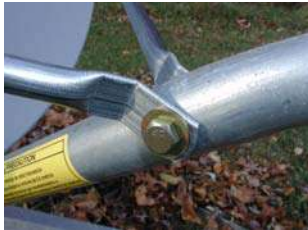
Support rod ends attached to feed support arm, in front of reflector
